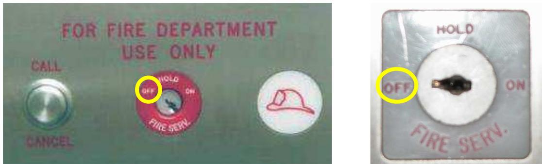
**Fig III: Turning the Phase II key switch to “OFF” will return the elevator car to the lobby.**
