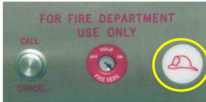
**A blinking helmet lamp indicates smoke or fire has been detected in the elevator hoistway or machine room.**
