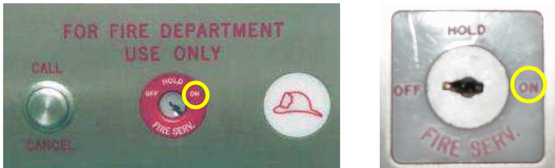
**Fig II: Phase II Elevator Key Switches**
