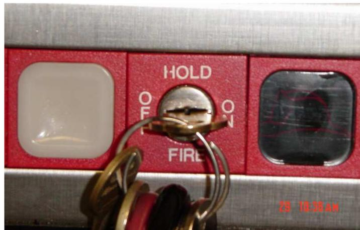
**Fig II: Phase II Elevator Key Switches**
