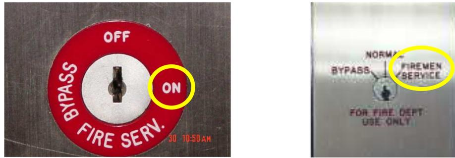
**Fig I: Phase I Elevator Key Switches**
